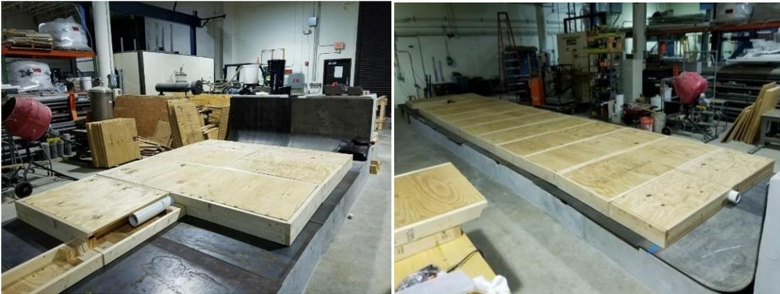
**Figure 82. Plywood boxes that form the refractory.**
